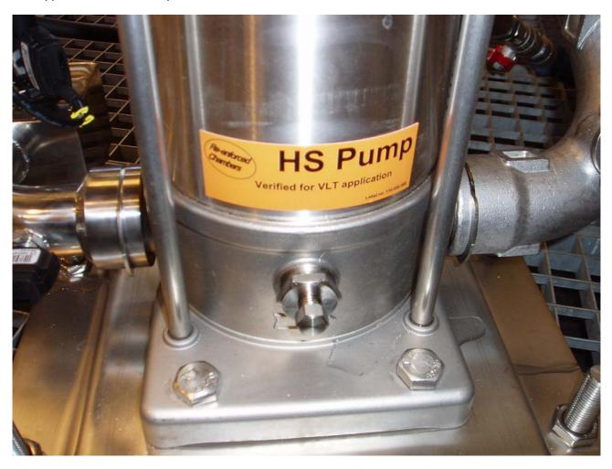
Also all spare part pumps and pump columns will be equipped with this label, showing that the pump is with reinforced chambers.
