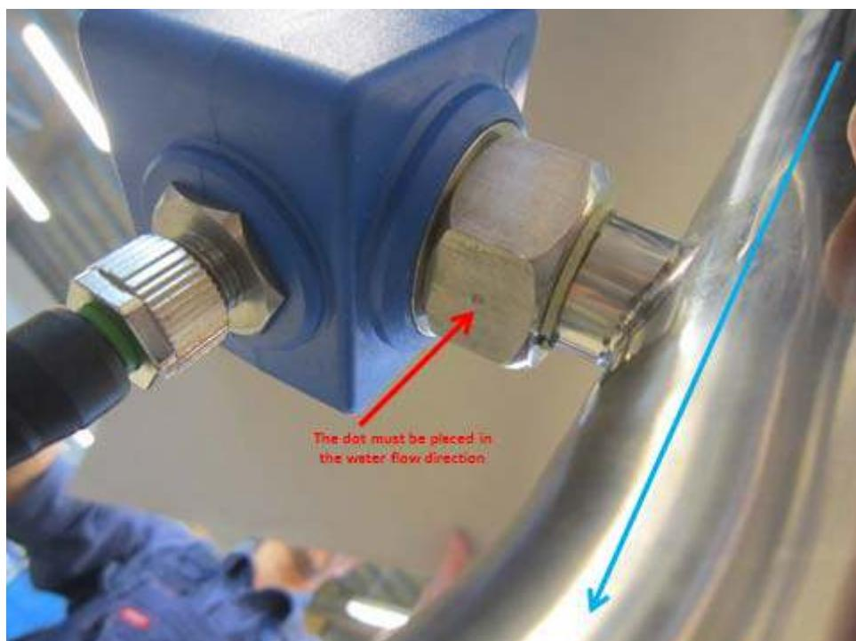
Please make sure that the flow switch is mounted in this way, in order to avoid that the flow switch shows flow even when there is no flow.
